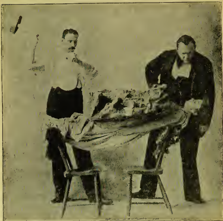
ROCK BREAKING TEST.
